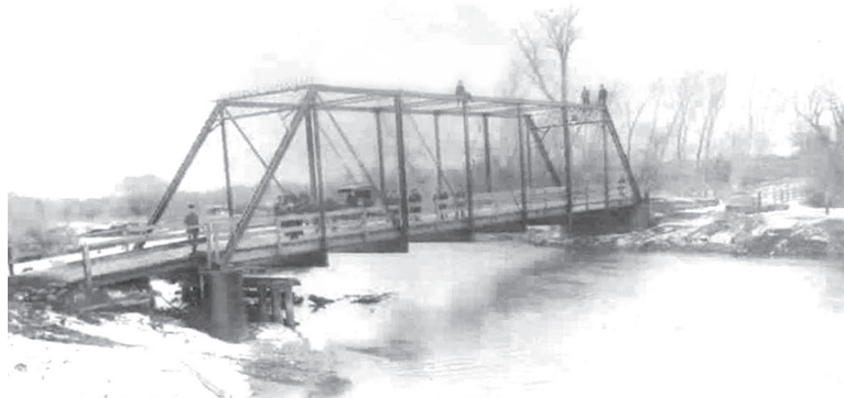
Bridge over Grande Ronde River at Orodell
