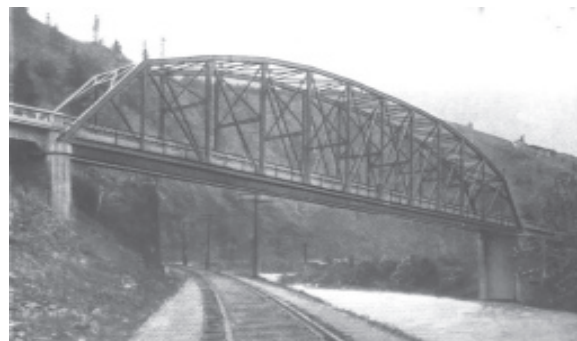
Old Oregon Trail (Highway 30) bridge over Grande Ronde River & Union Pacific mainline tracks, west of La Grande (demolished in early 1960s)
